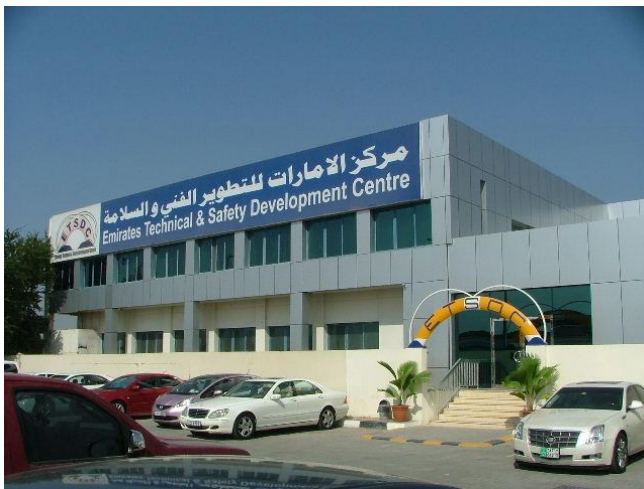
The Emirates Technical & Safety Development Centre in Mussafah, Abu Dhabi
